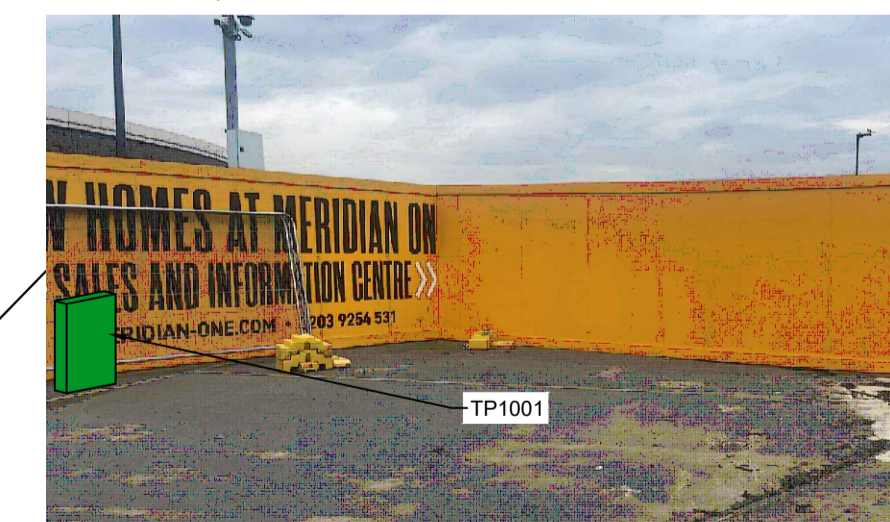
TP1001 Albany Road/Meridian One Site Test Point Cabinet Location Map Co-Ordinates E. 535065.628 N. 192131.221
