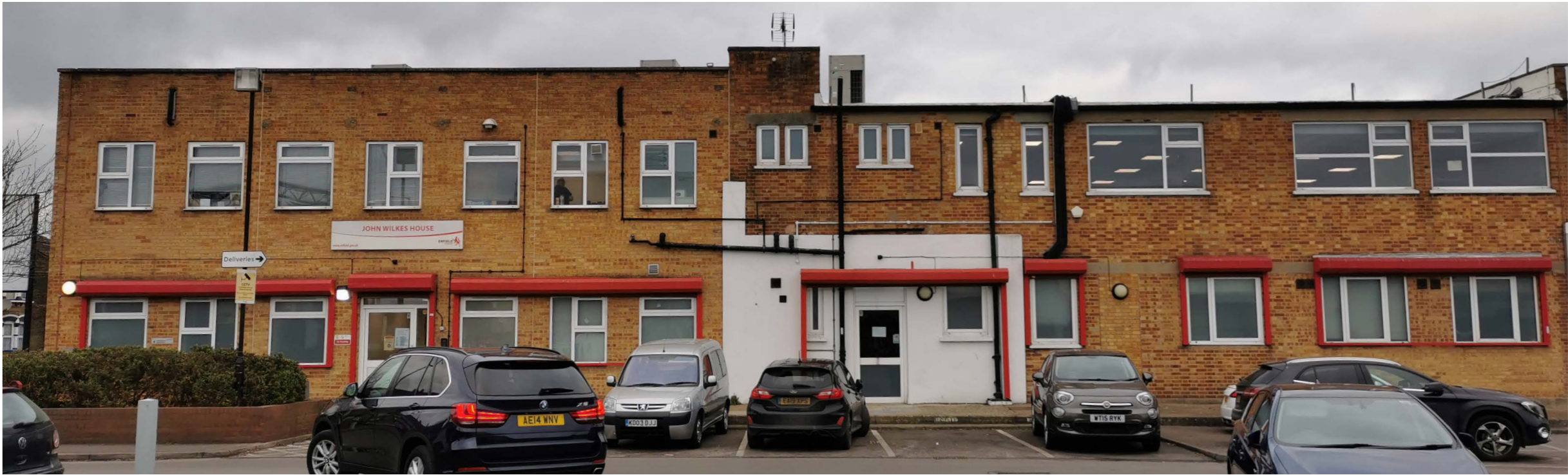
Part south elevation - shutters raised
