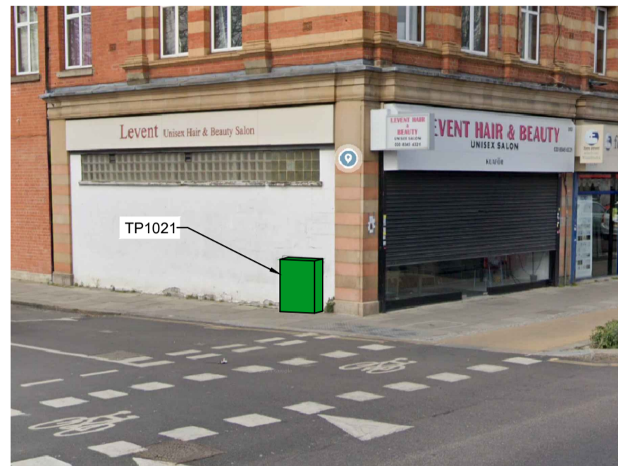
TP1021 Fore Street/Shrubbery Road Test Point Cabinet Location Map Co-Ordinates E. 534264.255 N. 193177.281
