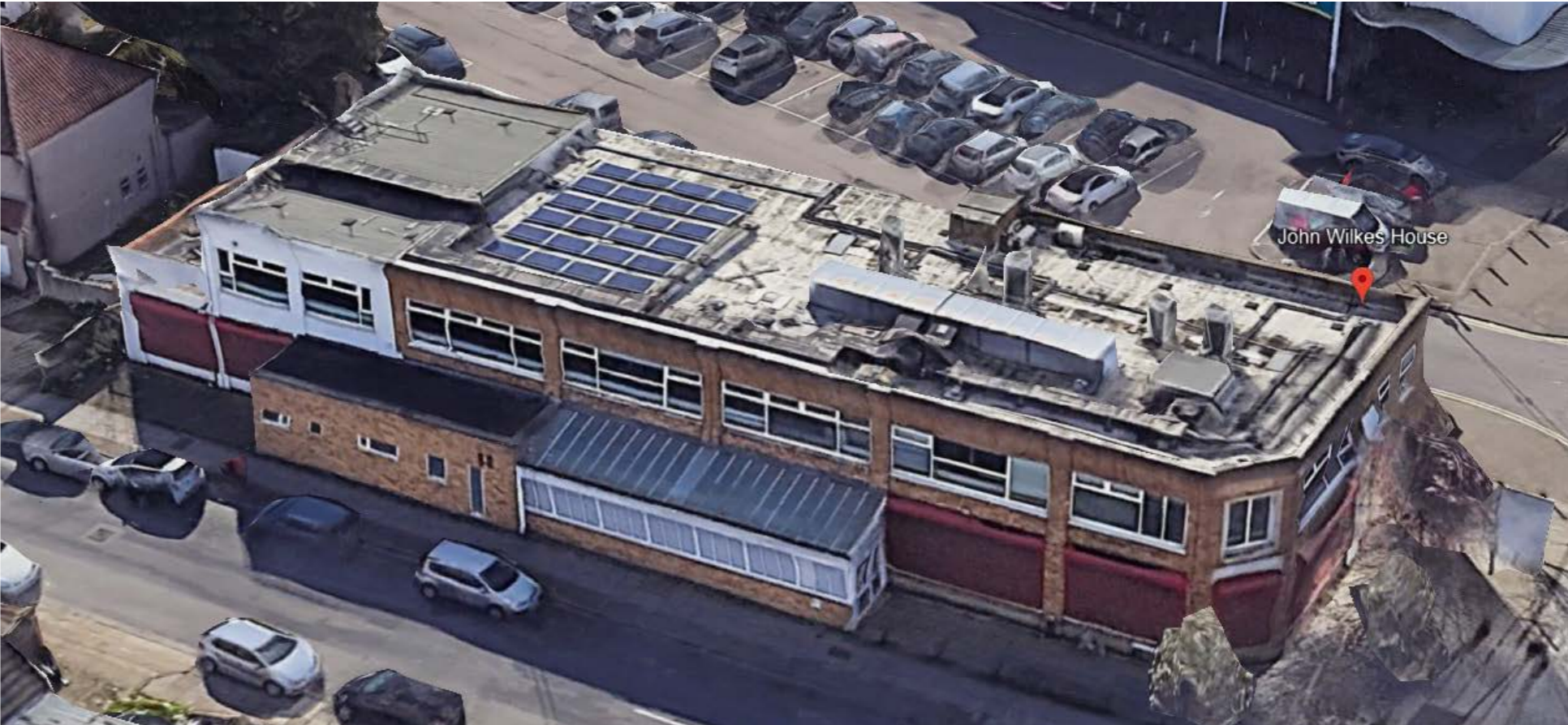
View from the North West
