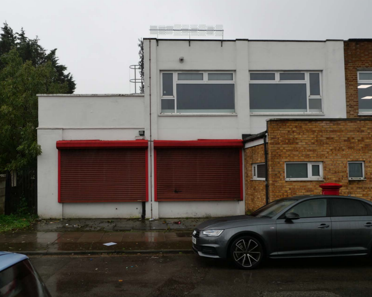
North elevation to Orchard Road
